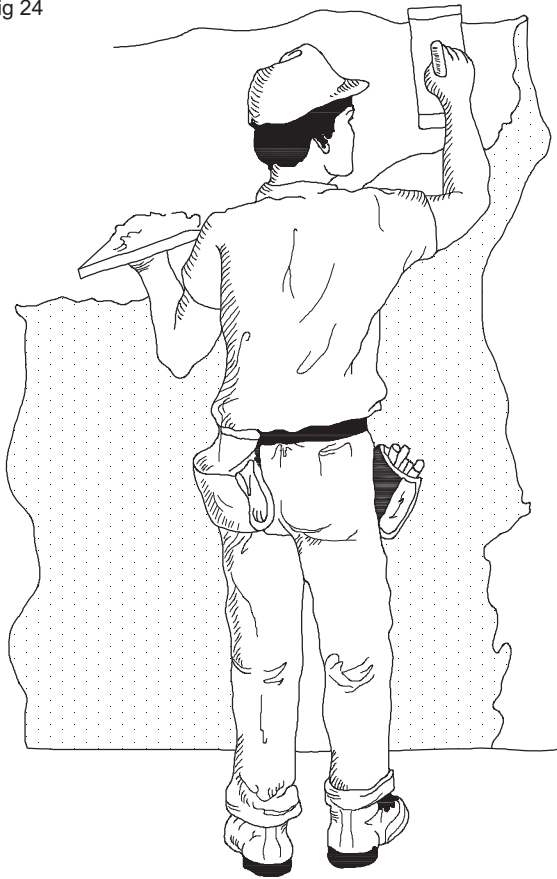
HOW PLASTER IS APPLIED TO THE WALL SHOWING THE USE OF THE HAWK AND THE TROWEL
